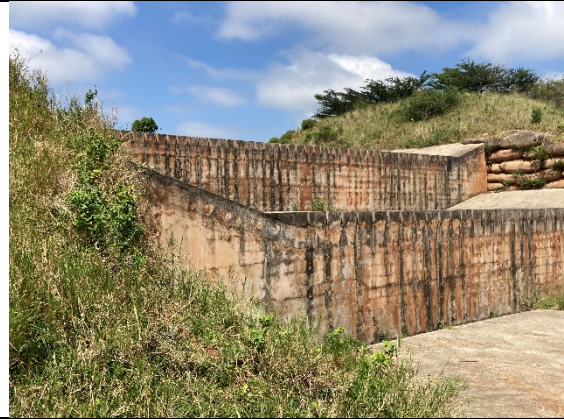
RSF spillway which is well maintained and fit for purpose.
